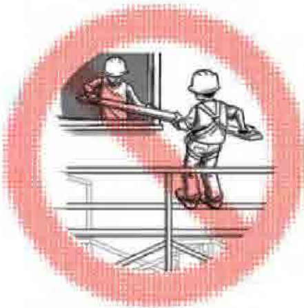
DON'T stand on guardrails
